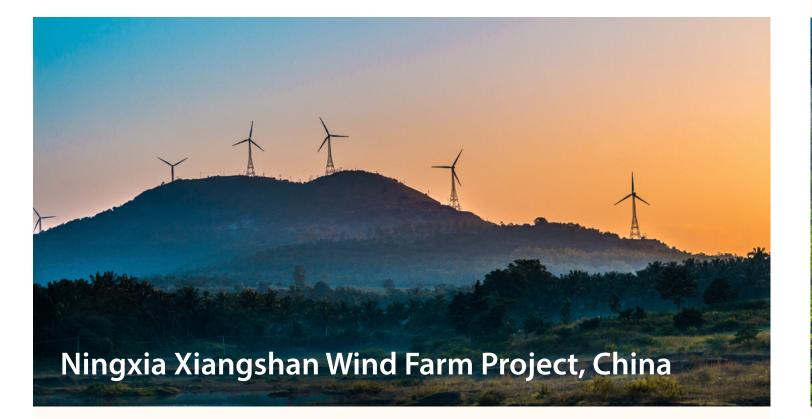
The project has a total installed capacity of 397.5MW consisting of 265 wind turbines with unit capacity of 1,500kW. The expected annual power delivered to the grid is 970,432MWh. The power generated will be delivered to the Northwest Power Grid (NWPG) via Ningxia Power Grid.
