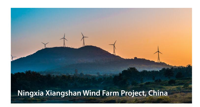
The project has a total installed capacity of 397.5MW consisting of 265 wind turbines with unit capacities of 1,500kW. The expected annual power delivered to the grid is 970,432MWh. The power generated will be delivered to the Northwest Power Grid (NWPG) via Ningxia Power Grid.
